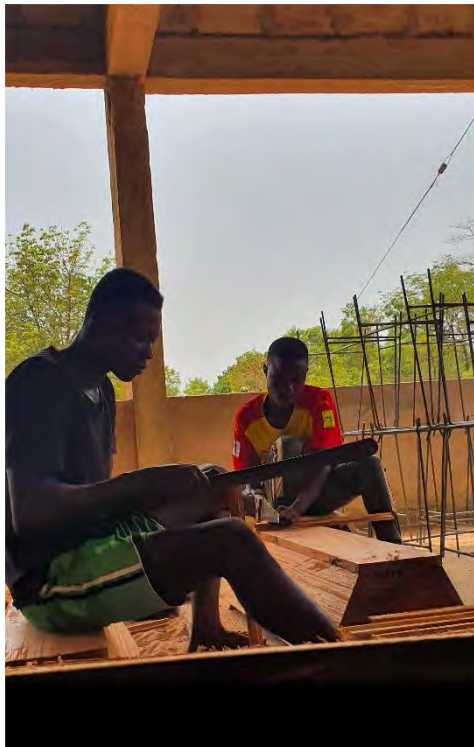
Preparing top bars
